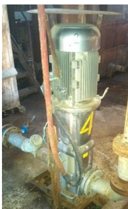
New pump for fresh water distribution
